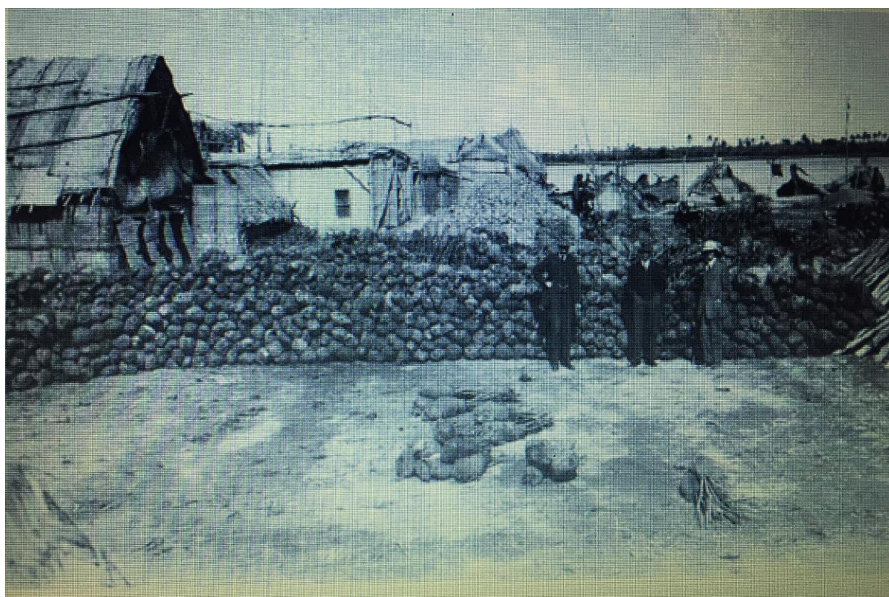
Figure 34: Shipment of date-palm offshoots from Basra to the U.S. in 1913. From Hopper, Slaves of One Master , 186.
